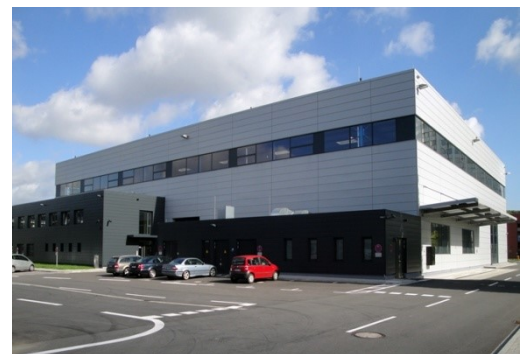
Fig.2: Production Site Mülheim
