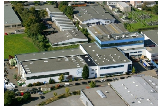
Fig.1: Main Plant Solingen
